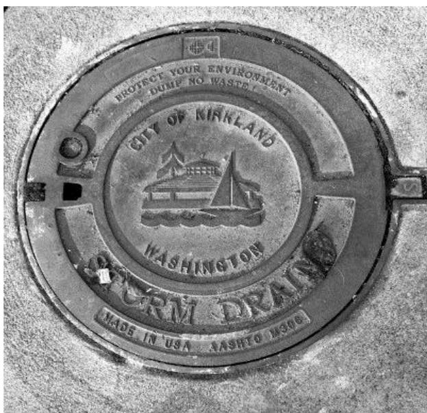
The answer to the pop quiz: Manhole covers are round so they can't fall into the hole they cover when tipped vertically (note that there is a small ledge that holds them in place, making the diameter of the hole slightly smaller than the diameter of the cover. If they were square, they could fall into the hole at a diagonal, or else the ledge would have to make the hole too small to get into, at least with the current size of holes—just big enough for workers to climb in and out.
